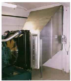
Under normal conditions, the air volume generated from the radiator's fan is enough to meet the requirement of the working room ventilation.
