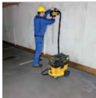
Certified extractor and dust extractor for extracting health hazardous dusts in accordance with EN 60335-2-69.
