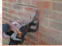
Cutting openings for windows / doorways
