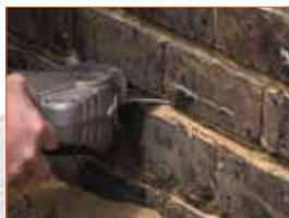
DPC, Cavity tray & wall tie replacement
