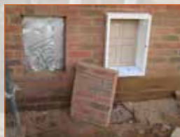
Cutting out for service boxes
