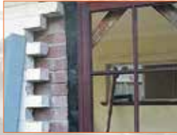
Toothing & bonding brickwork
