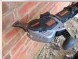
Repointing with minimal dust
