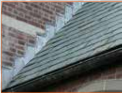
Raking out for lead flashings
