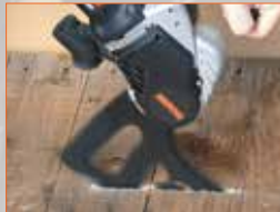
Cutting out floor boards
