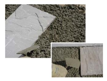
Always maintain at least a 3mm gap width throughout the depth of the paving material. This is particularly important when working with paving that has chamfered edges. See photograph below.
