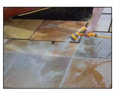
Once you have opened and spread one or two tubs, using a hose on a "fan" or "spray" setting, flush the compound into the joints to ensure it fully settles to the bottom. Again, do not worry about the amount of water being used. You can do this as often as you like—after each tub is fine. **Remember** - the wetter the better!
