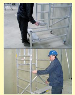
The steps and diagonal braces are fitted before the platform is placed in position.
