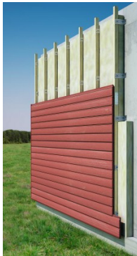
Cladding installation
